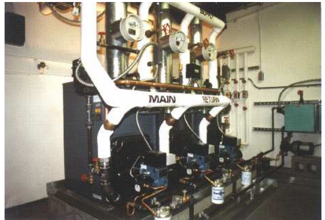
COMMERCIAL BUILDING – FAIRBANKS, ALASKA 1994
