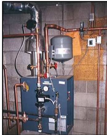
TYPICAL RESIDENTIAL BOILER AND HW HEATER INSTALLATION 1994 & 2003 - EAST & WEST ANCHORAGE
