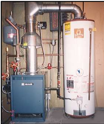
TYPICAL RESIDENTIAL BOILER AND HW HEATER INSTALLATION 1994 & 2003 - EAST & WEST ANCHORAGE
