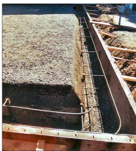
MONOLITHIC EDGE FORMS DESIGNED AND INSTALLED BY JERRY 1998
