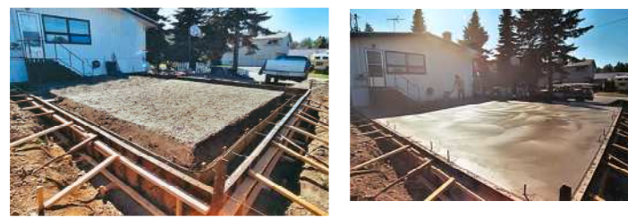
MONOLITHIC EDGE FORMS DESIGNED AND INSTALLED BY JERRY 1998
